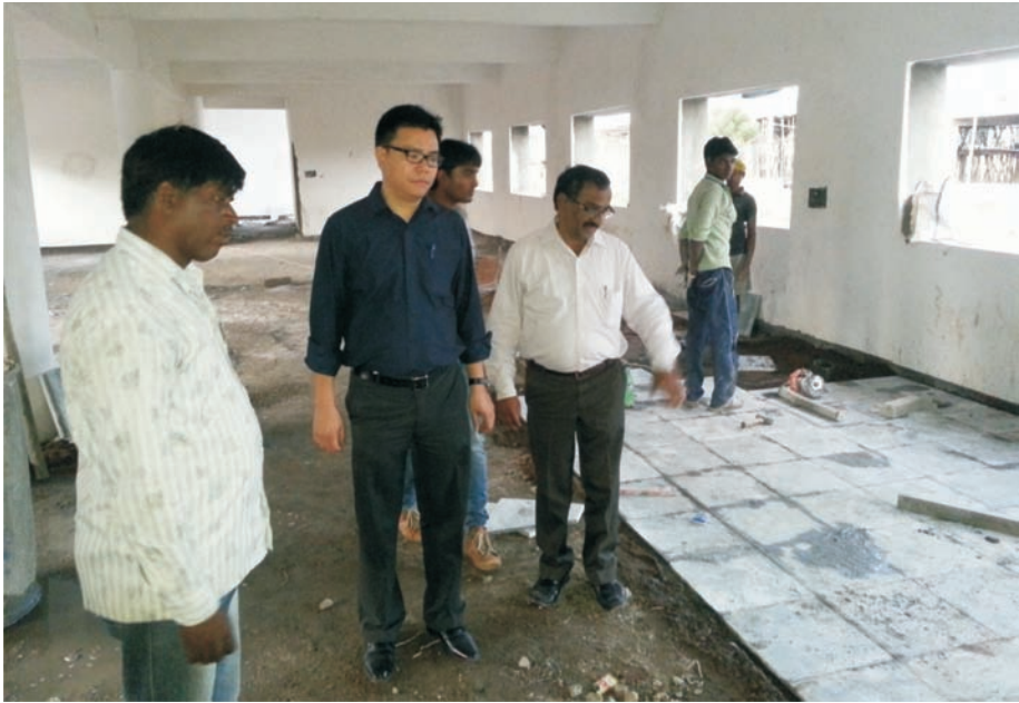
Observation of construction work at KGTTI, Gulbarga Centre
